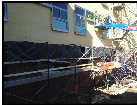
Bldg C East Façade – Windows & Brick
