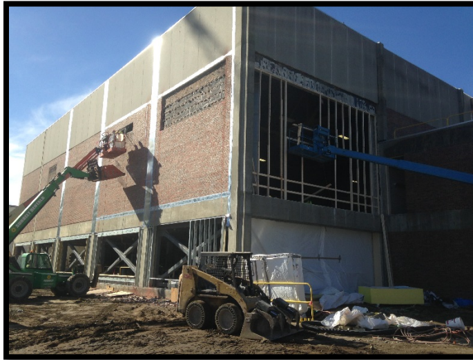
Building E Northeast Corner
