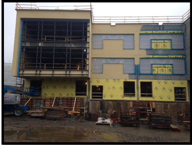
Bldg C North – Curtain Wall & Loading Dock
