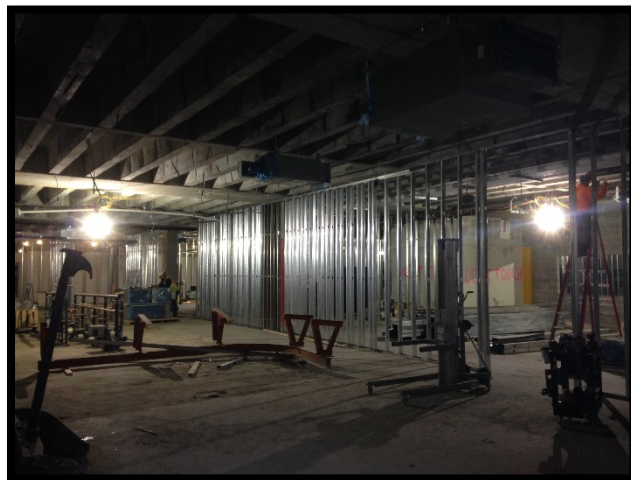
Bldg E Level 1 – Framing
