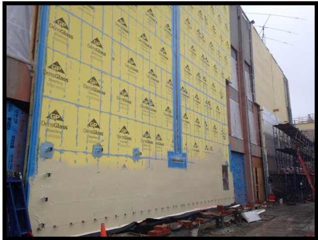
Bldg E South – AVB & Brick
