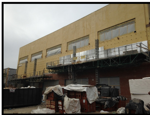
Bldg E East – Brick Installation
