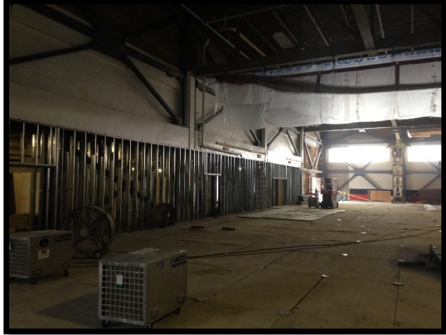
Bldg E Level 2: Steel Bracing and Framing
