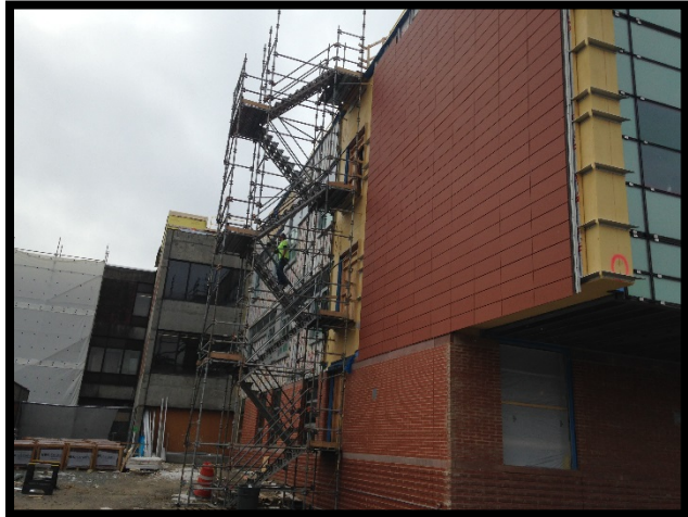
Bldg C East – Terracotta & Arriscraft Install
