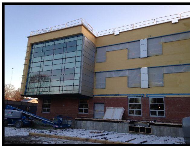
Bldg C North – Metal Panel and Window Install
