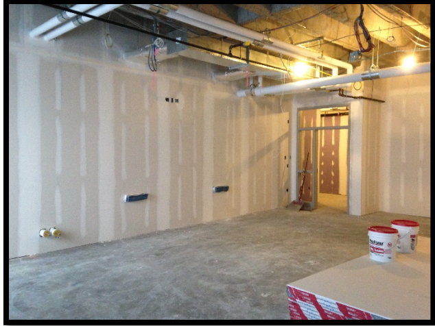
Bldg C: Drywall/Taping Classrooms
