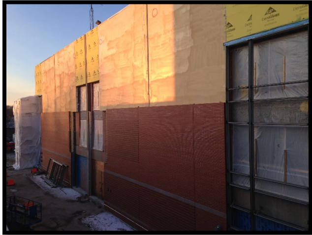
Bldg E South – Curtain Wall and Brick Install
