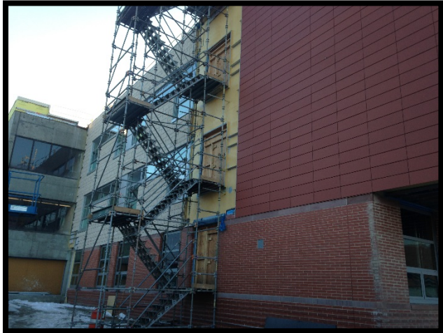
Bldg C East – Arrsicraft and Terracotta Install
