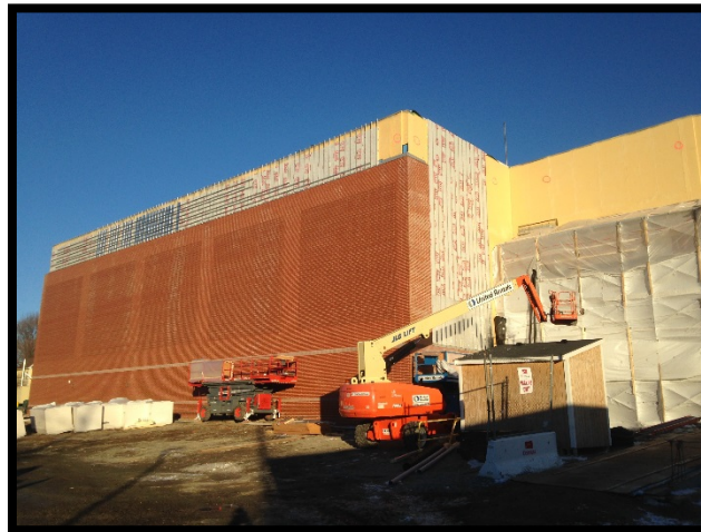
Bldg E West – Arriscraft and Brick Install
