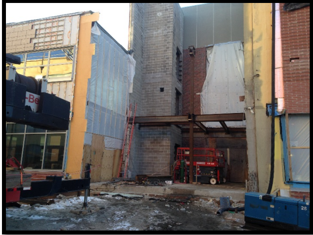
Bldg D/E Connector: Steel Erection
