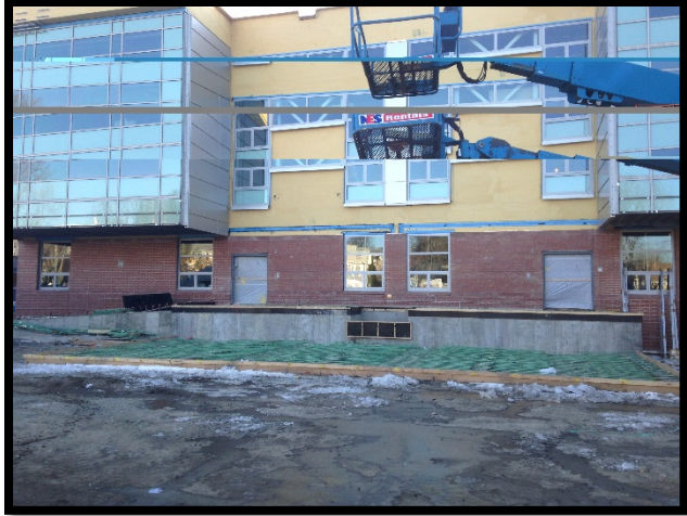
Bldg C North – Loading Dock Slab Prep
