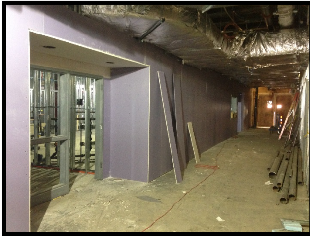
Bldg E Level 1: Drywall Install
