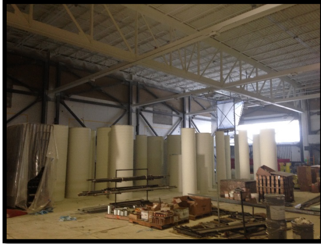
Bldg E Level 2 – Painting Overhead Spiral Ductwork
