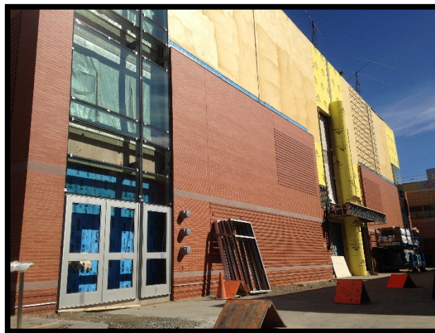
Bldg E South – Curtain Wall, Arriscraft, & Canopy Install
