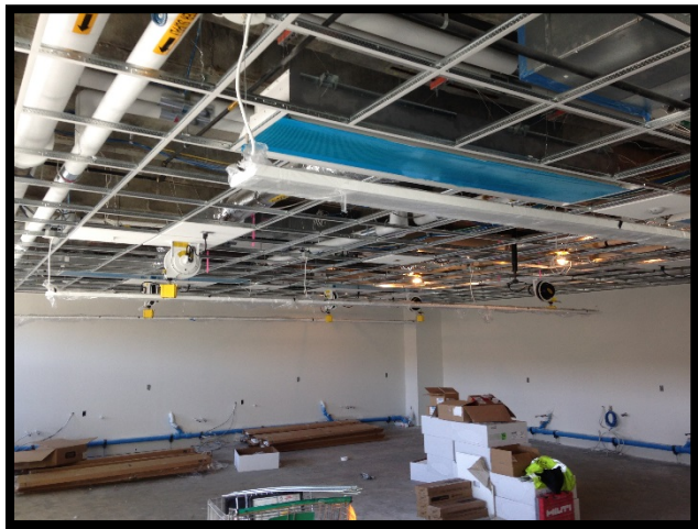
Bldg C Level 3 – Light Fixture & Cord Reel Install
