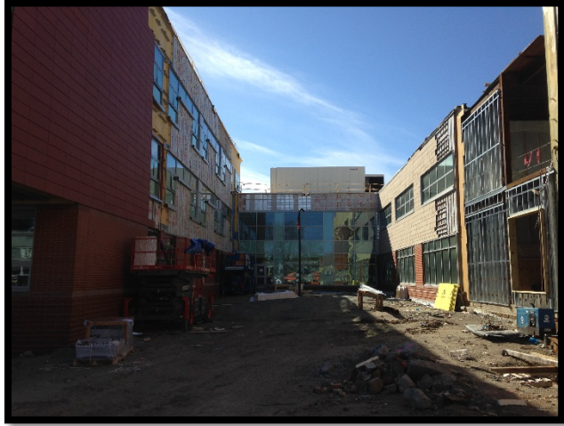
Bldg C/E Courtyard: Exterior Framing & Arriscraft Install
