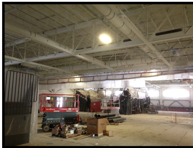
Bldg E Level 2 – Overhead MEPs & Painting
