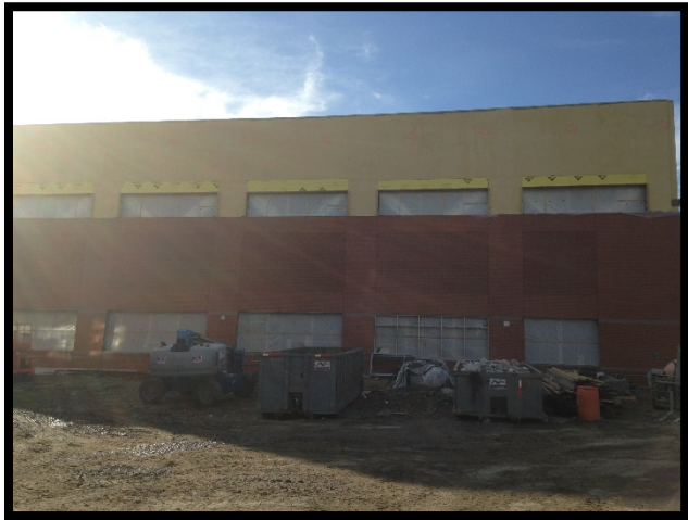
Bldg E East – Exterior Window Install
