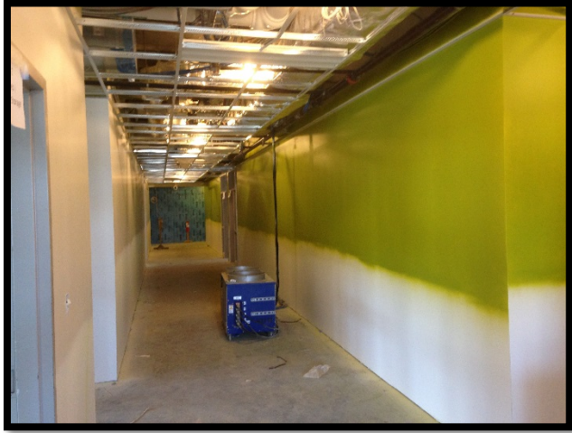
Bldg C Level 2: Corridor
