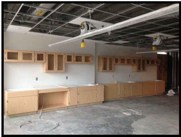
Bldg C Level 3 – Casework Install
