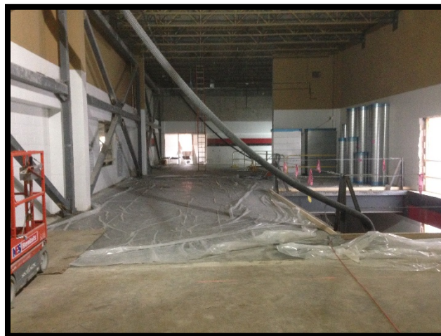
Bldg E Level 2 – Mezzanine Infill Concrete Placement
