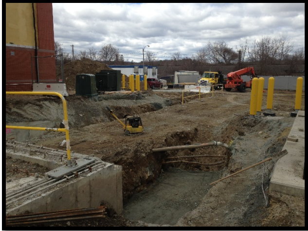
Bldg E – Retaining Wall Excavation
