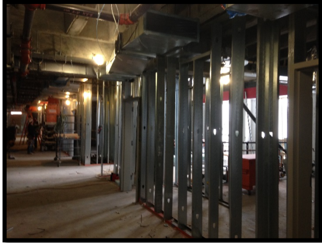
Bldg E Level 2 – Interior Framing
