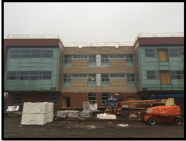
Bldg C North Veneer Installation
