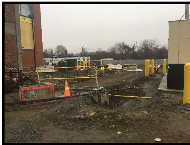
Bldg E Retaining Wall
