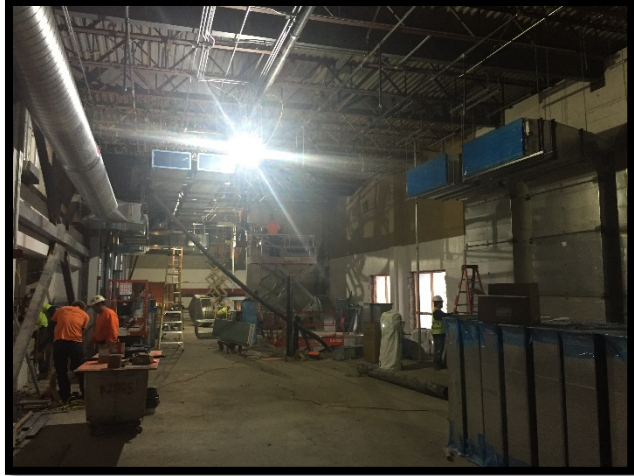
Bldg E 3 rd Floor – MEP Installation
