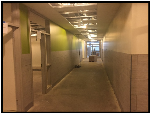
Bldg C 3 rd Floor - Tile Installation
