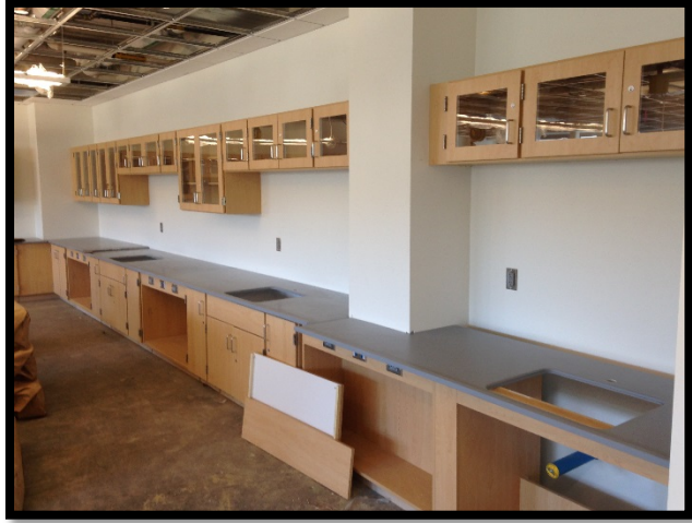
Bldg C 3 rd Floor – Countertop Installation
