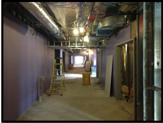
Bldg E Level 2: Overhead MEP & Framing
