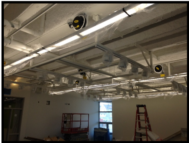
Bldg C 1 st Floor – Fixture Installation
