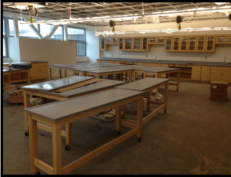
Bldg C Level 3 – Classroom Casework
