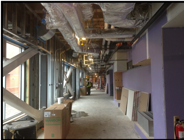
Bldg E Level 1: Overhead MEP Work
