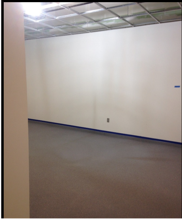
Bldg E Level 1: Resinous Flooring Install
