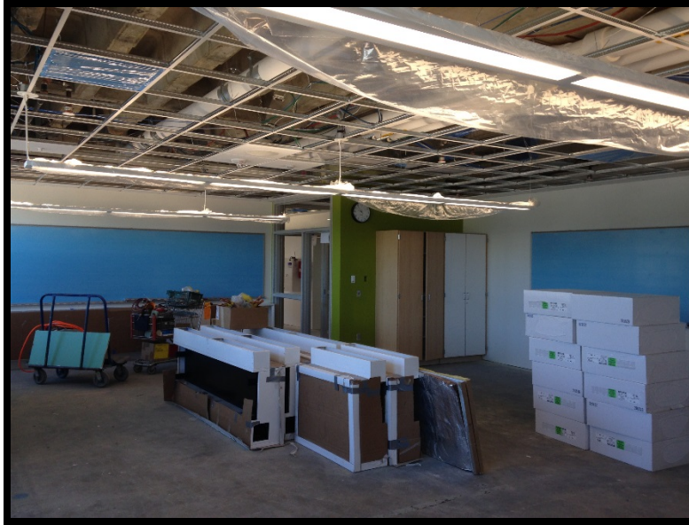
Bldg C Level 3 – Marker Boards & Radiators
