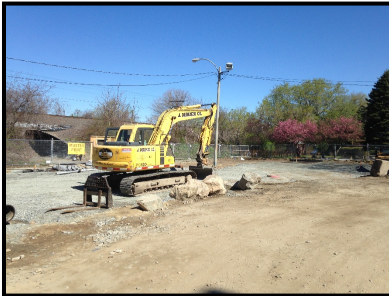
NW Corner: Grading for Temp Parking
