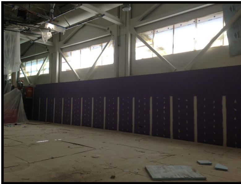
Bldg E Gym: Drywall/Tape Paint Low Walls
