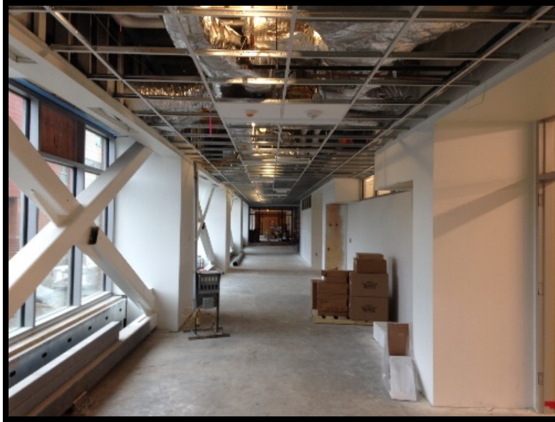
Bldg E Level 1: East Corridor
