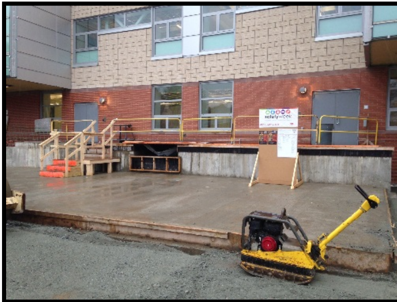
Bldg C North: Loading Dock Slab & Grading
