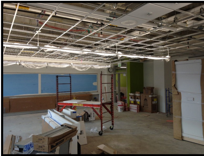
Bldg C Level 1: Ceiling Grid
