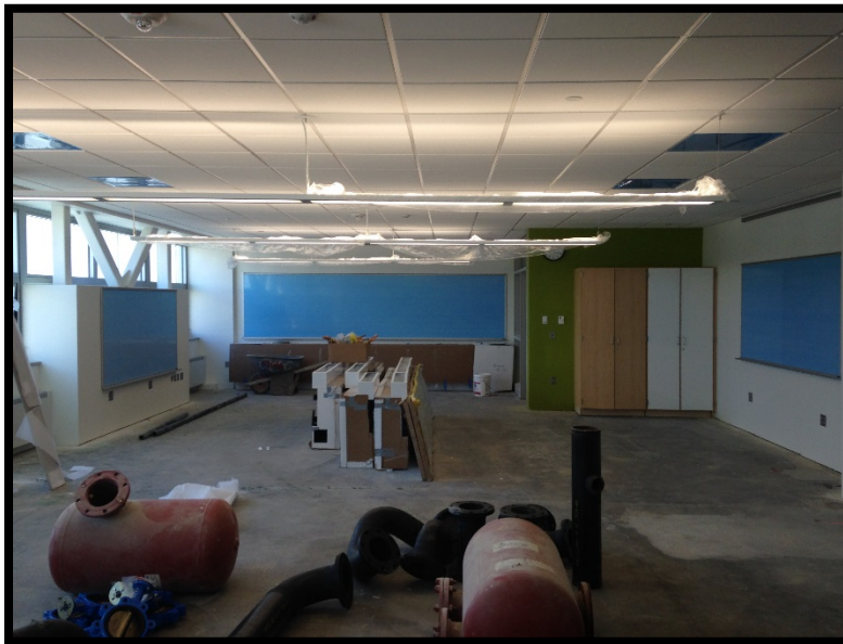
Bldg C Level 3: Markerboards
