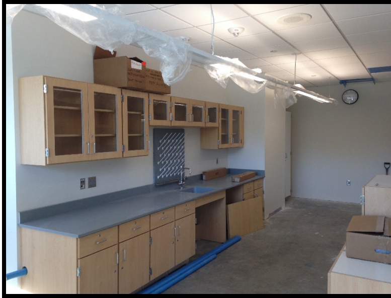
Bldg C Level 2 – Lab Prep Room
