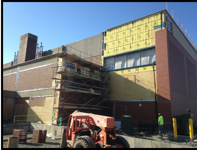
Bldg E Northwest: Brick & vapor barrier
