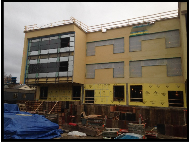
Bldg C North – Curtain Wall, AVB, and Loading Dock
