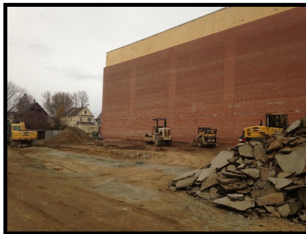
Bldg E West – Site Grading
