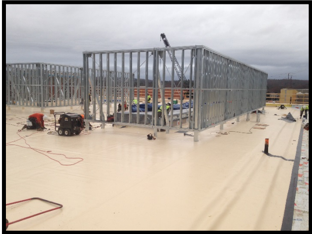
Bldg C Roofing
