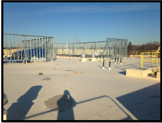
Bldg C PVC Roof Completion
