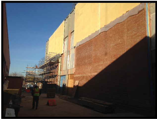
Bldg E South – Brick Installation
