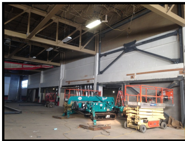
Bldg E Level 2 – Interior Structural Steel Erection
