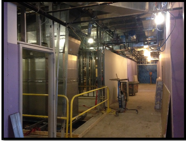
Bldg C Level 2: Drywall Install & Mechanical Shaft Work
