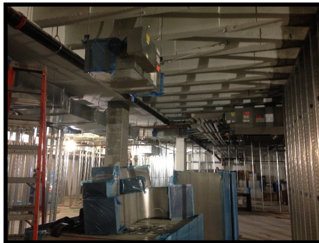
Bldg E Level 1 – Interior Framing and Overhead MEP Work
