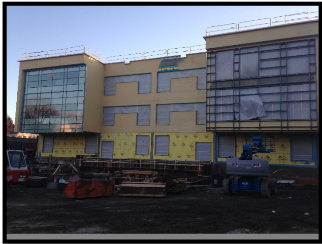
Bldg C North – Curtain Wall & Concrete Work
