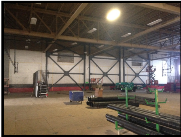
Bldg E Level 2 – Steel Erection & Overhead MEP
