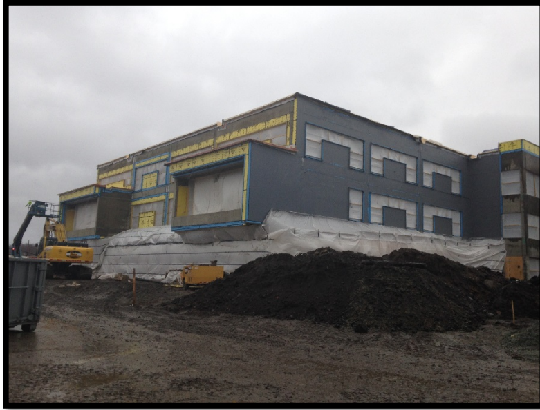
Bldg A South/East: Brick Veneer & AVB
