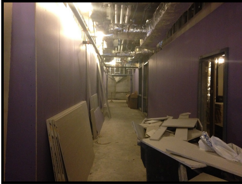
Bldg B Level 2: Drywall Installation
