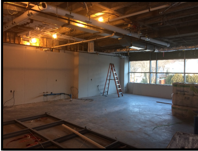
Bldg B: Physics Lab at 2 nd Floor
