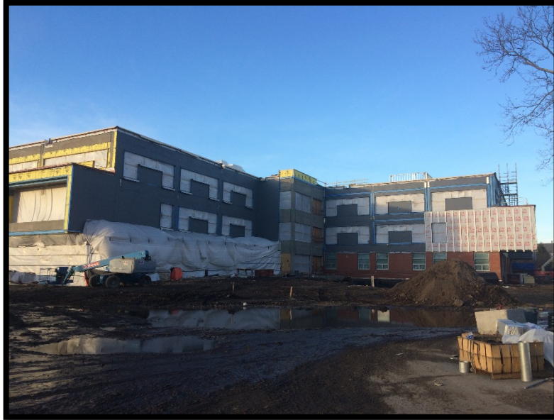
Bldgs A & B: Installation of Exterior facades ongoing
