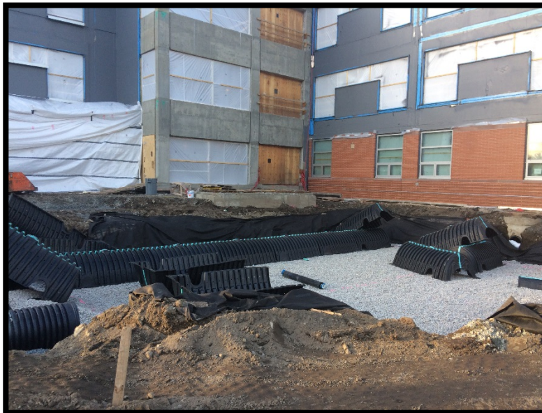
Site: Installation of water filtration system ongoing
