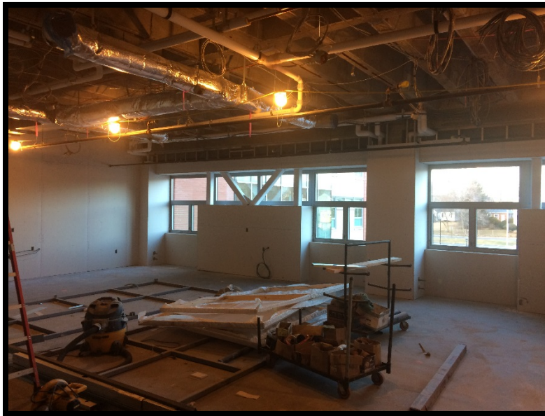
Bldg B: Typical Classroom at 3 rd Floor
