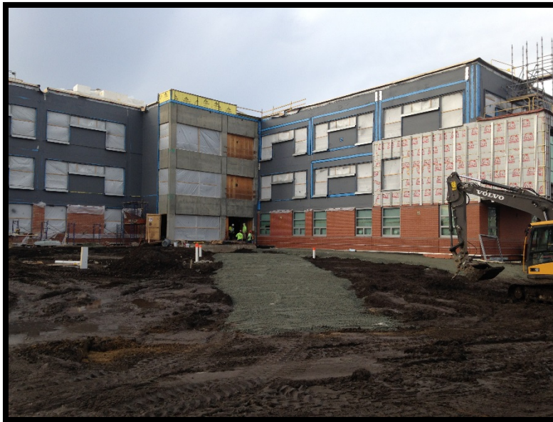
Bldg A/B Courtyard: Grading & Recharge System Installation
