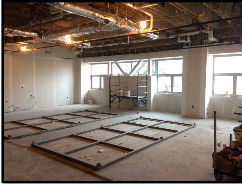
Bldgs B Lvl 2: Taping/Mudding & Pipe Grid Install
