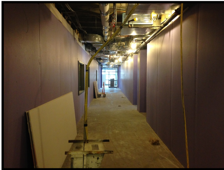
Bldg B Lvl 3: Drywall Install in Corridors
