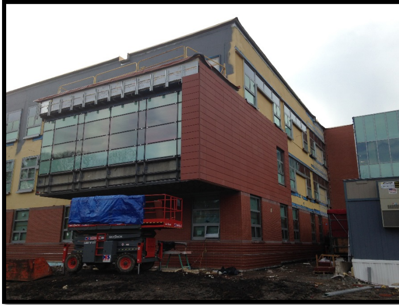
Bldg B North: Terracotta & Arriscraft Installation
