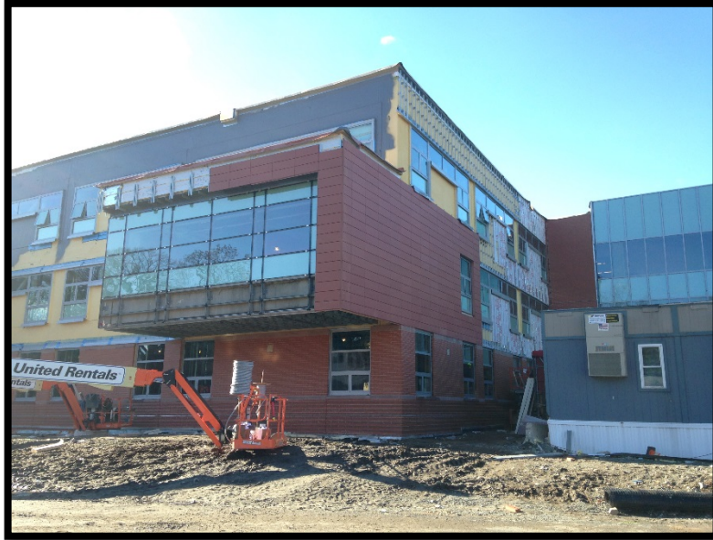
Bldgs B North: Terracotta & Arriscraft Installation
