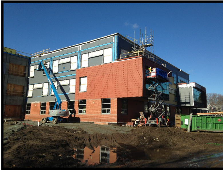
Bldg B South: Terracotta & Window Installation
