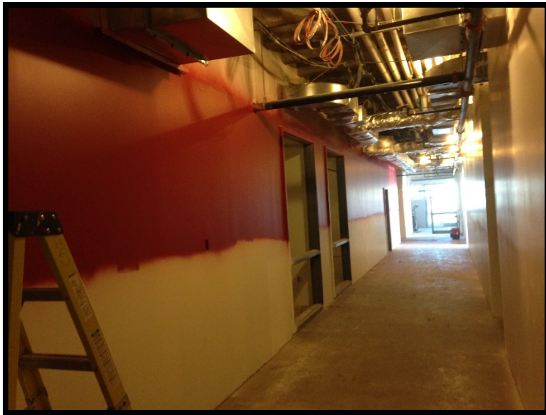
Bldg B Lvl 2: Painting
