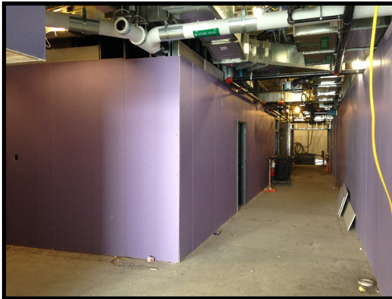
Bldg A Lvl 2: Drywall Installation
