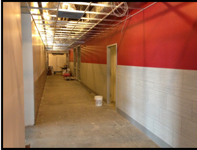
Bldg B Lvl 2: Corridor Tile
