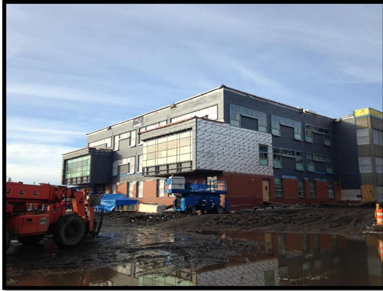
Bldg A South/East: Terracotta & Curtain Walls
