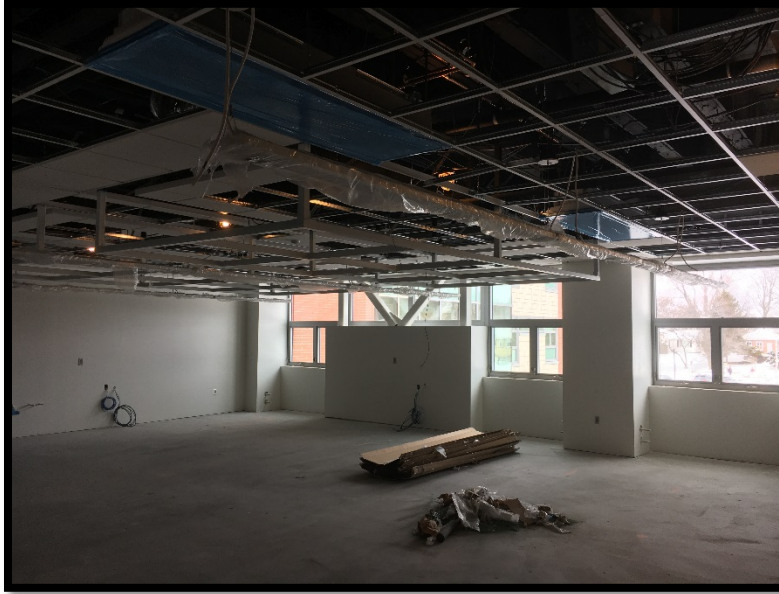
Bldg B Lvl 2: Ceiling Grid & Fixtures in Classrooms
