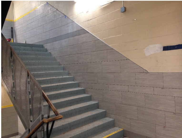
Bldg B Lvl 2/3: Tile Stairwells
