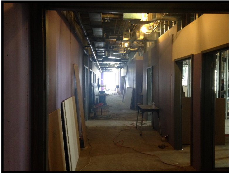
Bldg A First Floor: Drywall Installation
