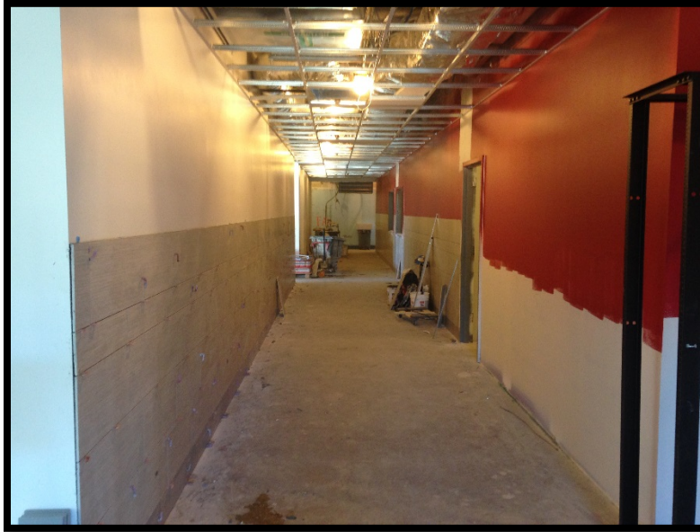
Bldg B Lvl 3: Ceiling Grid & Corridor Tile
