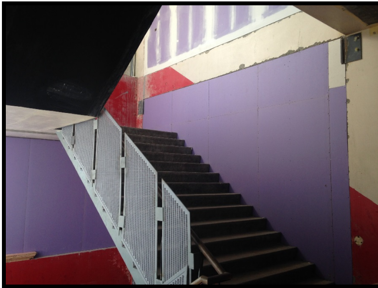
Stair A: Drywall & Perforated Panels
