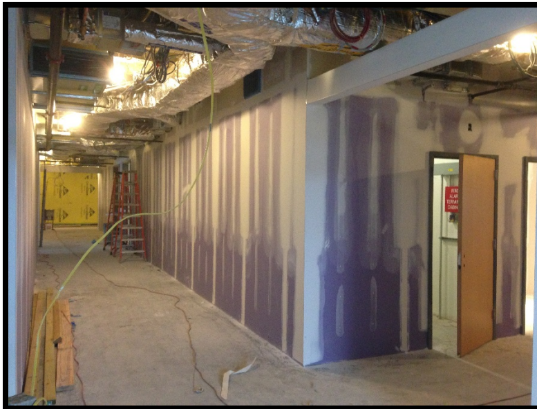
Bldg A Lvl 3: Mudding & Taping
