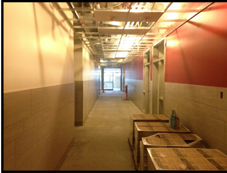
Bldg B Lvl 2: Corridor Tile & Painting Complete
