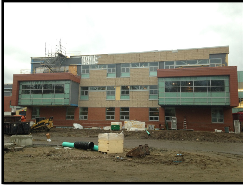
Bldg B East: Arrsicraft Complete
