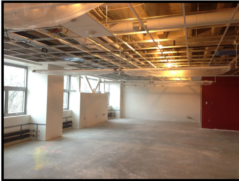
Bldg B Lvl 3: Ceiling Grid & Fixtures
