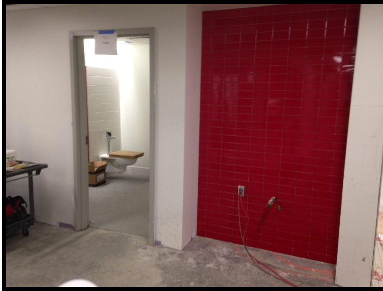
Bldg E Level 1: Corridor & Bathroom Tile
