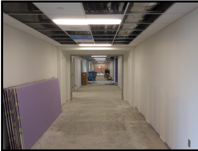
Bldg E Level 2: South Corridor
