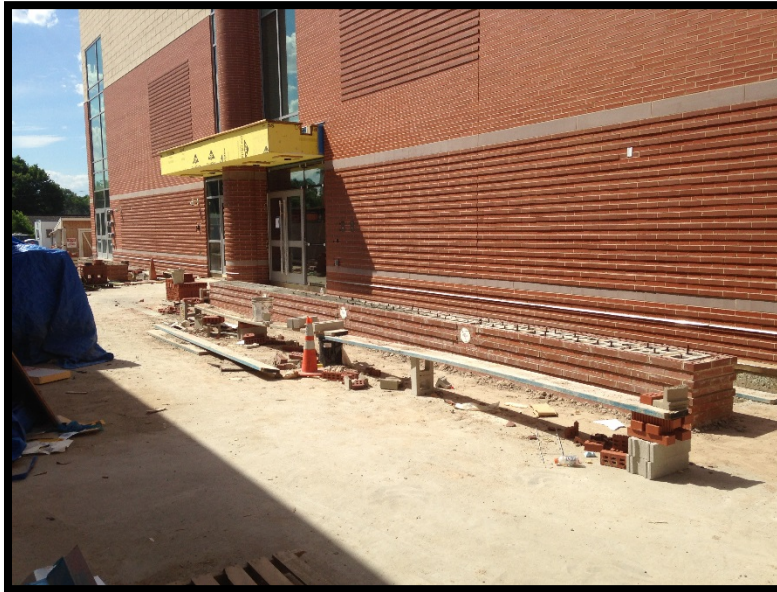
Bldg D/E Plaza: Brick Planter Install
