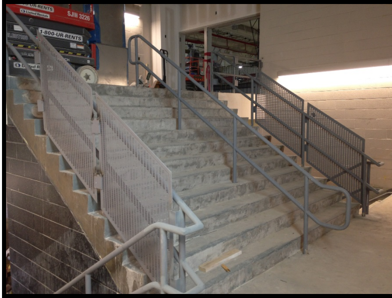
Bldg E – Railings Install
