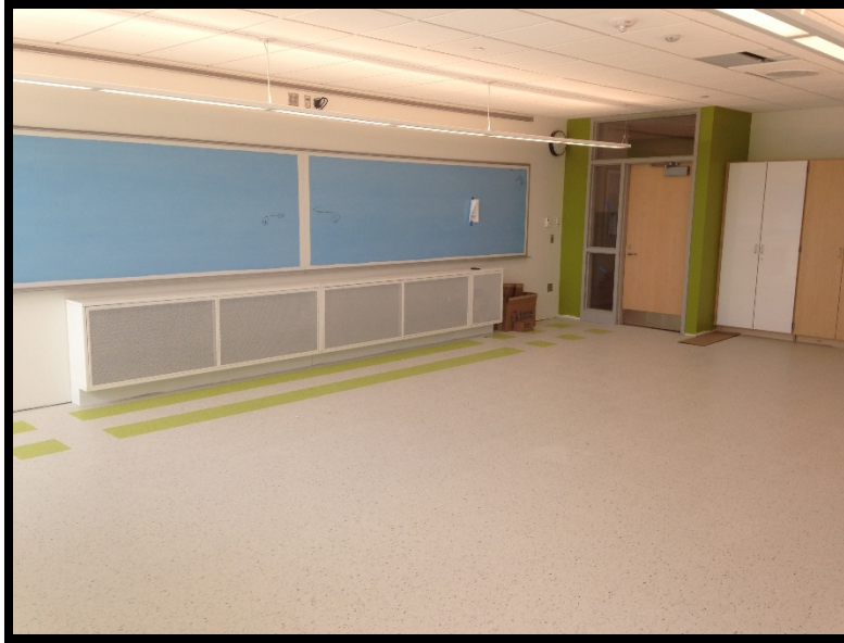
Bldg C Level 3: VCT Flooring
