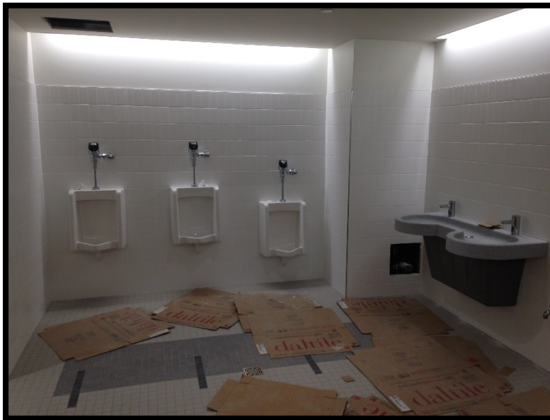
Bldg E Level 1: Plumbing Fixtures
