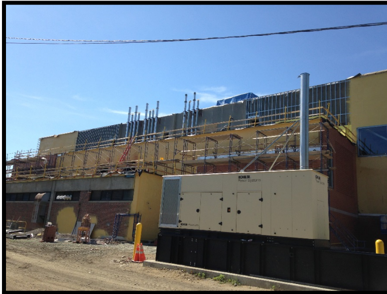
Bldg E North: Framing & Brick Veneer
