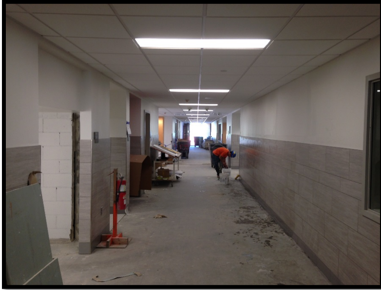
Bldg E Level 1– South Corridor
