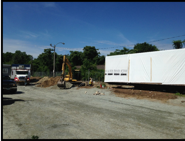
West Side of Site: Construction Trailer Removal & Excavation
