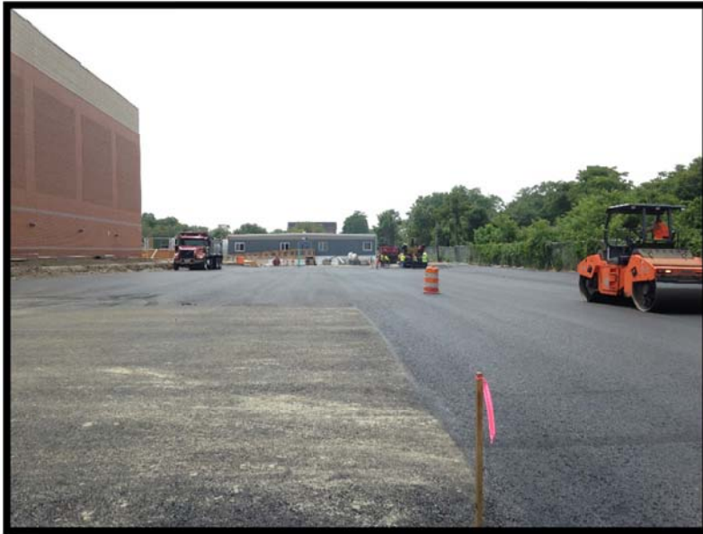
West Side of Site: Paving for Phase 3 Modular Classrooms
