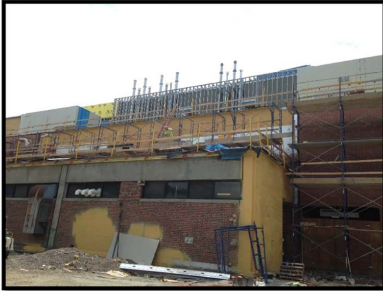
Building E North: Exterior Framing & Brick Install
