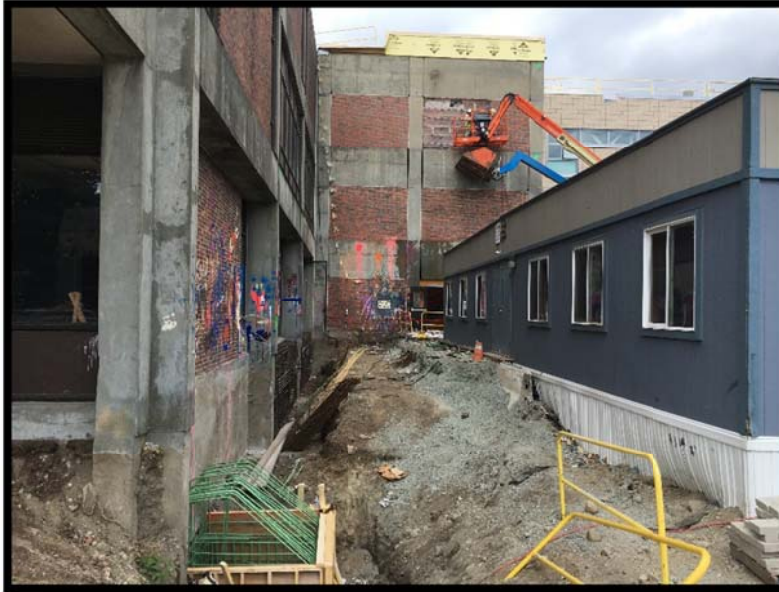
Bldg B North: Demo of Stair C & Grade Beam Install
