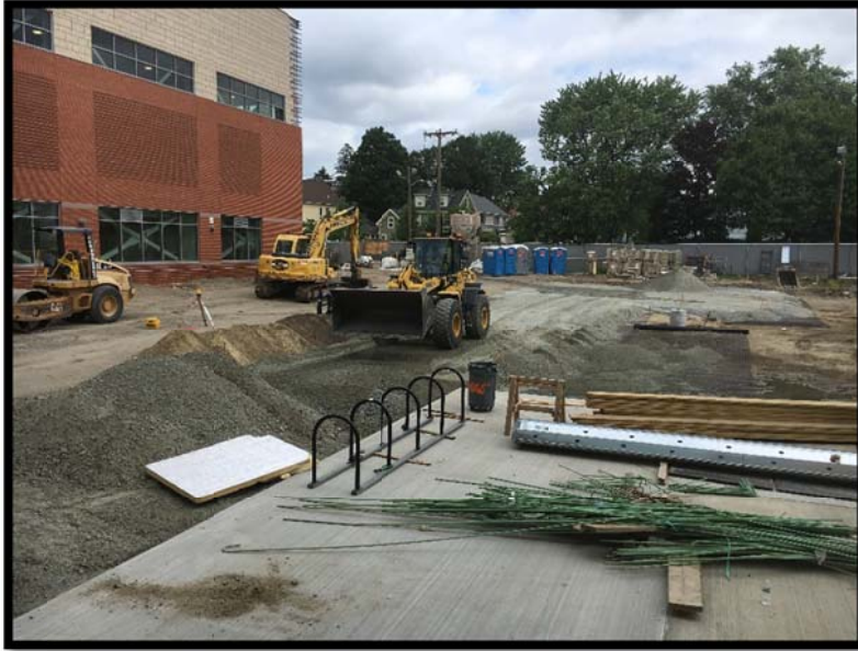
Building E East: Grading & Site Prep
