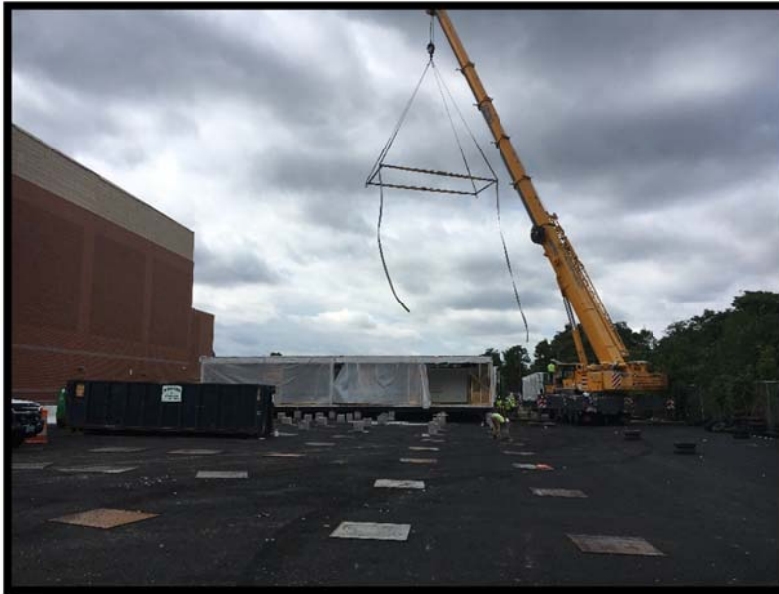
West Side of Site: Setup of Phase 3 Modular Classrooms
