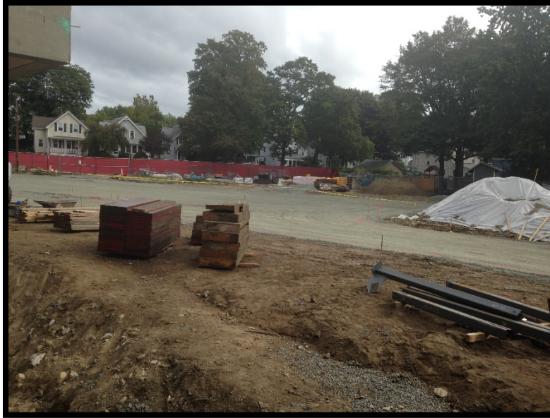
Northeast Corner: Prep for Paving
