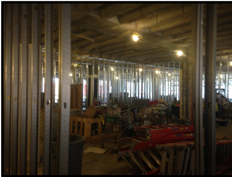
Bldg B: Interior Framing
