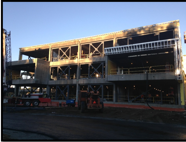
Bldg A South: Exterior Framing & Bracing
