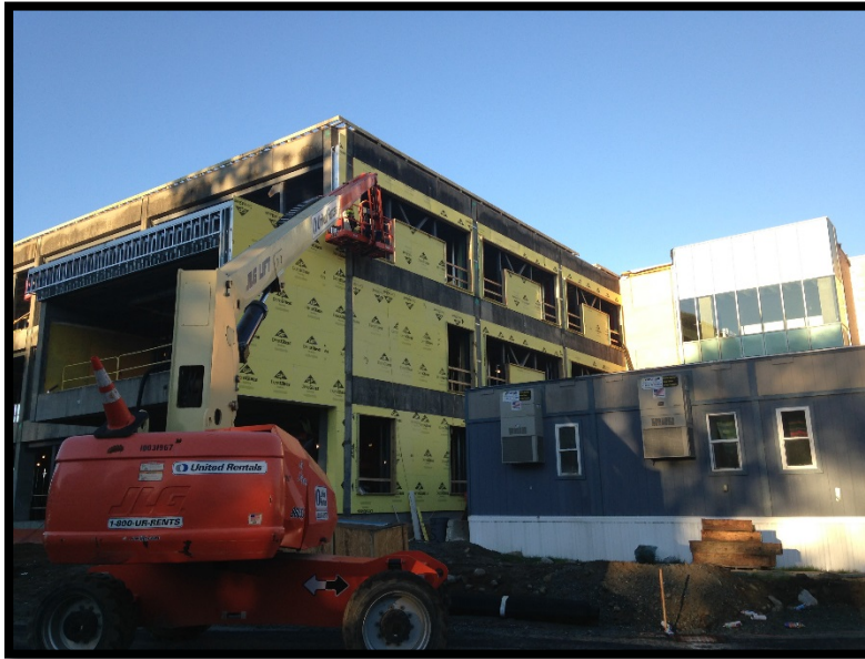
Bldg B North: Exterior Sheathing
