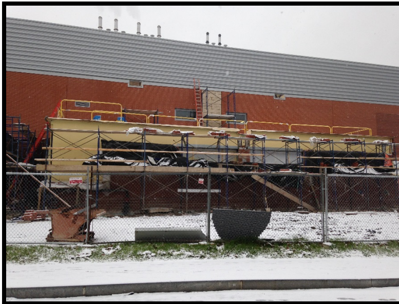
Bldg E North: Brick Installation
