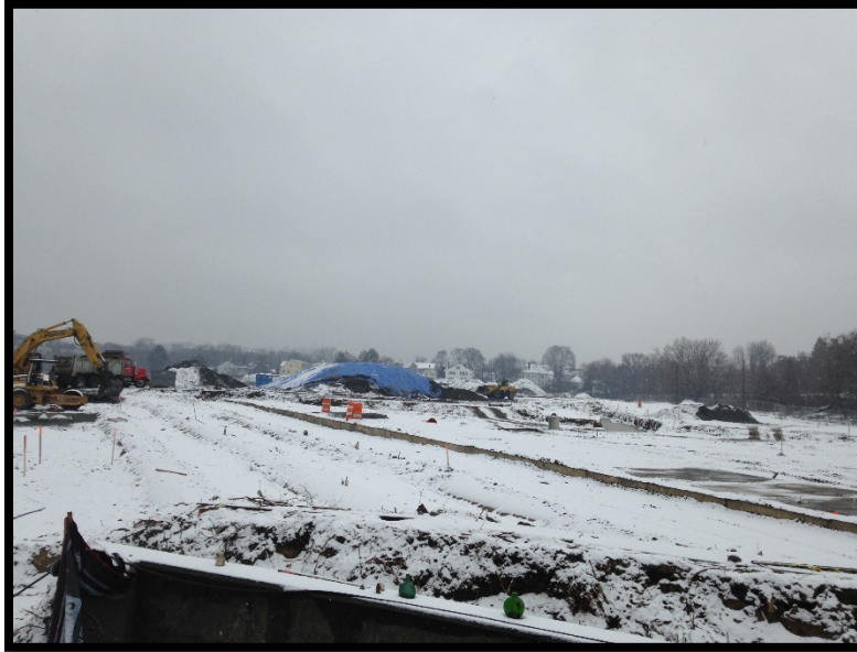
Skillings Field: Prep for Culvert Fabric Cap
