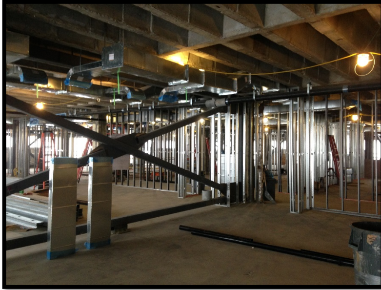
Bldg A Lvl 3: Interior Framing & Mechanical Rough
